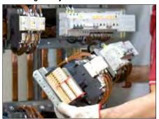
In case of breakdown the plates (the system's main characteristic) can be easily replaced with new ones of the same type with a very simple operation.
