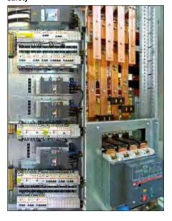
The control panel has been designed so that no live part can come into contact with the operator's body even with the main door open, according to the degree of protection IP XX B of standard IEC 529.
